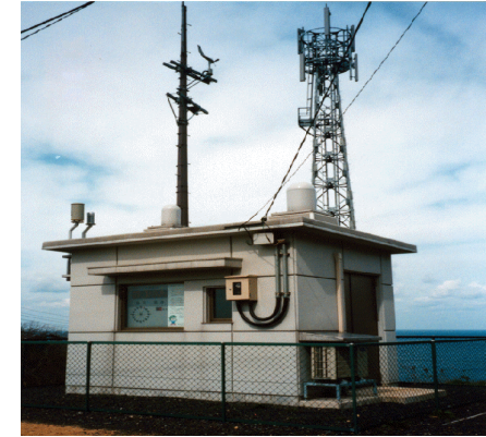
Air-monitoring station in Japan
