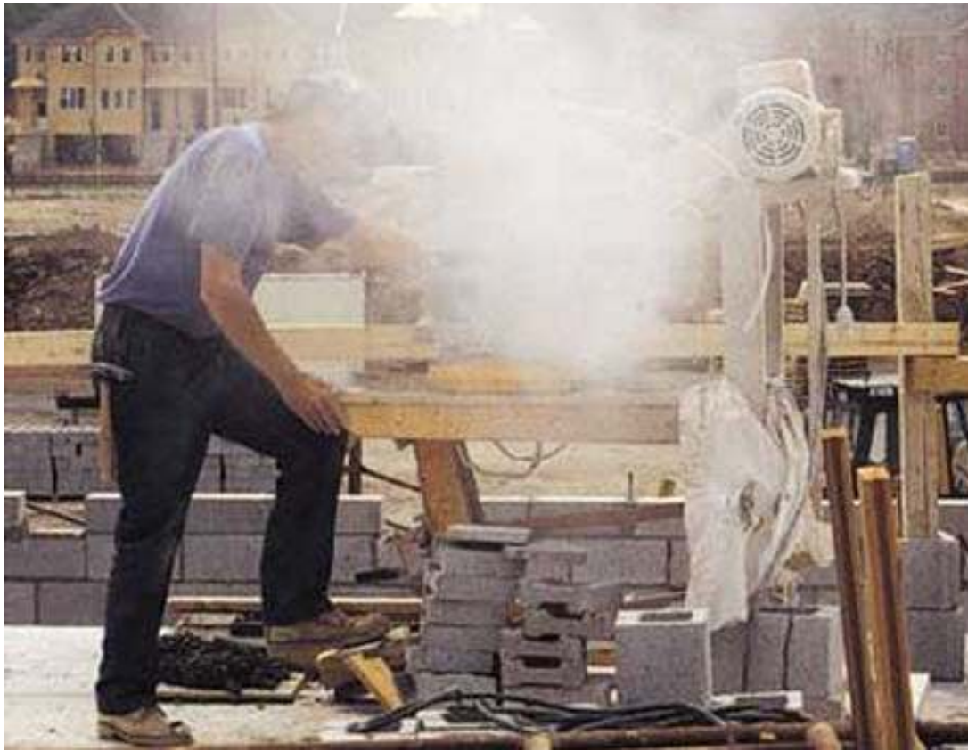
Dry cutting stone...
